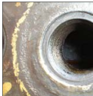
Plug hole before re machining the gasket seat
