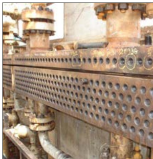
FinFan cooler before a maintenance
