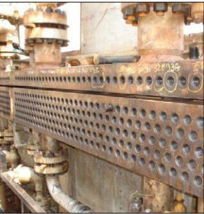
FinFan cooler before a maintenance
